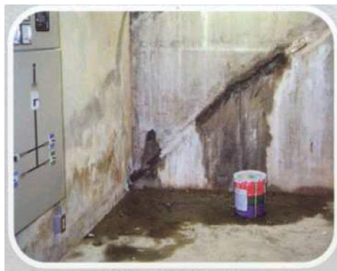
Fisura reparata in a doua zi
